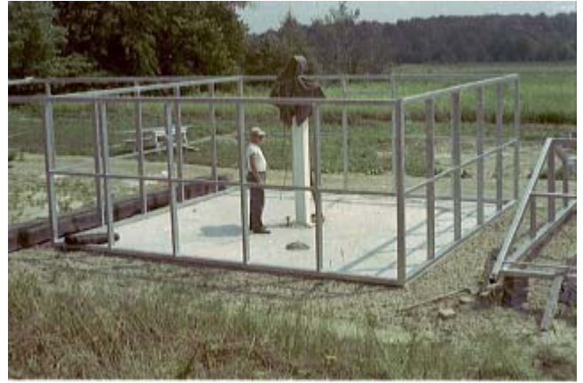
Above: The steel framework for the 8" building takes shape.
